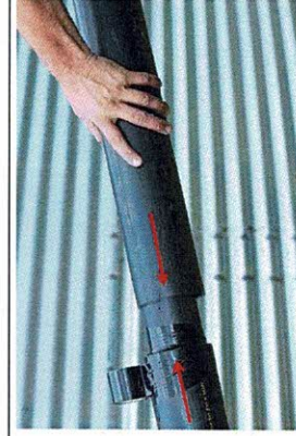
1. Buis verbinding/pipe connection
