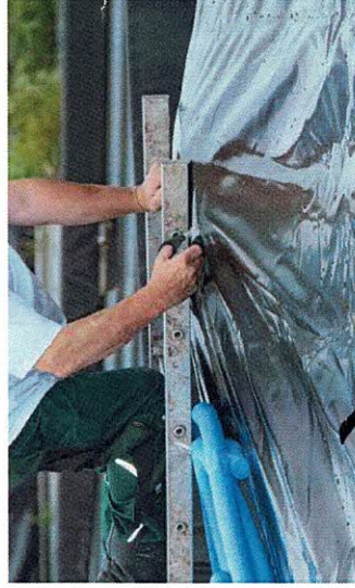
Opening in zeil knippen / cut opening in cover
