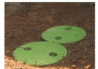
Last 20 – 30 cm of the pit bury with the earth.
