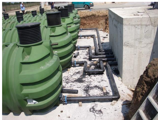
Picture 7: Foundation slab
