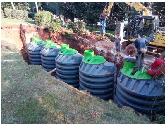
Picture 5: Installed tanks in a row
