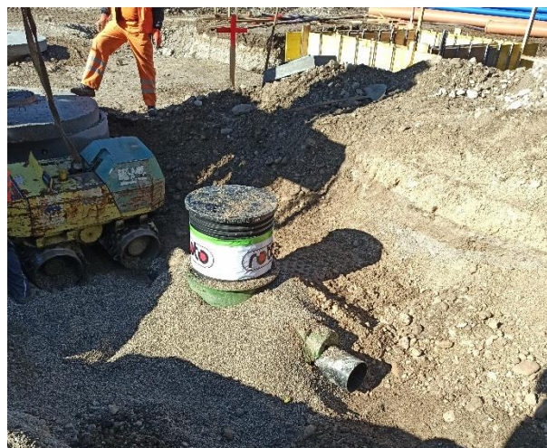
Picture 8: Burry of the reservoir with 4 – 16 mm
