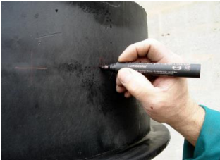
Mark the place of the inflow pipe (PE shaft has straight surface for inflow)
