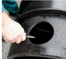
Clean the borehole
