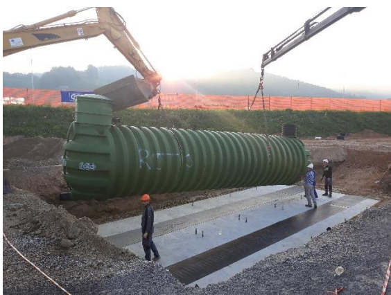
Picture 4: Installing the tank
