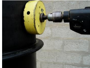
Drill the inlet borehole with a suitable crown drill
