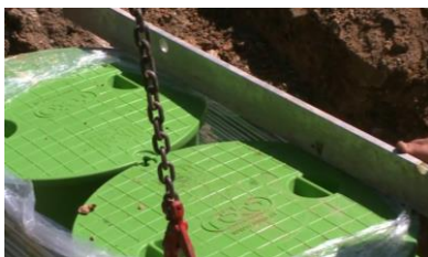
Make sure that the cover and the terrain are correctly leveled out
