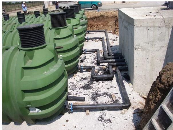
Picture 7: Foundation slab
