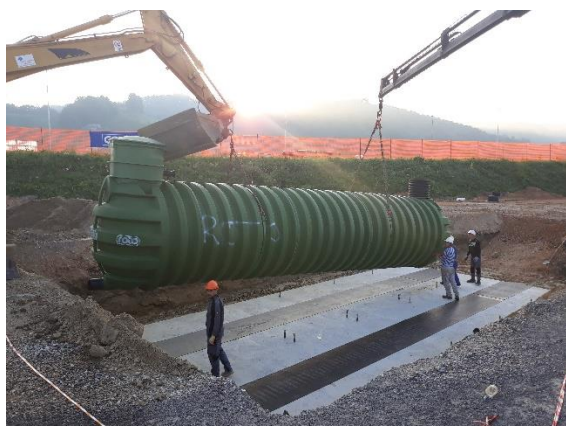
Picture 4: Installing the tank
