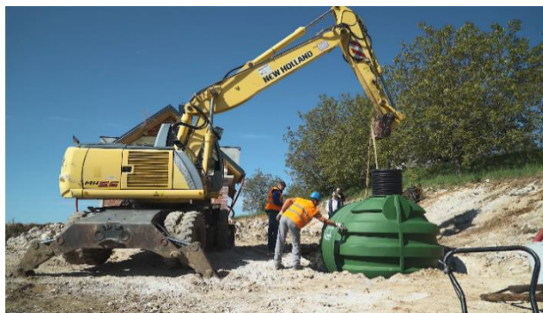
Picture 3: Installing the tank
