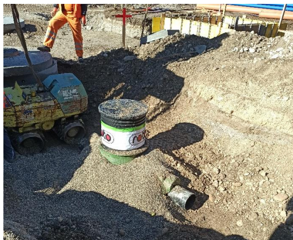
Picture 8: Burry of the reservoir with 4 – 16 mm
