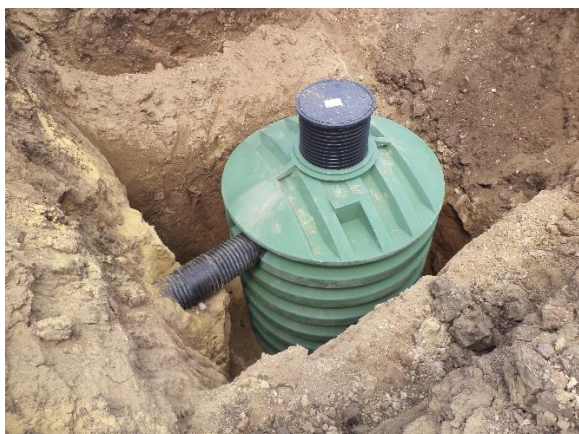
Picture 6: Installed tank
