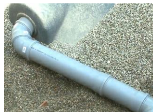
Carefully bury the pumping station with the correct gravel of 4 – 16 mm granulation
