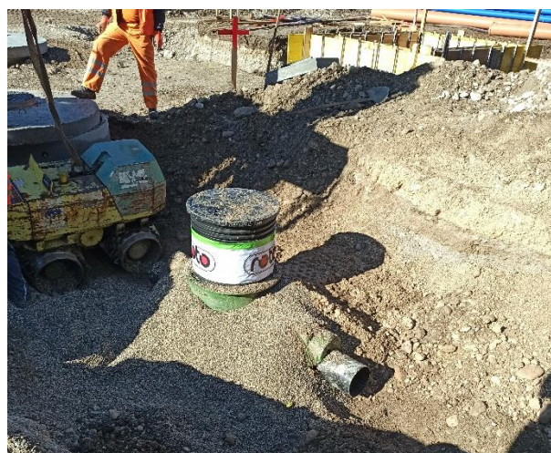
Picture 8: Burry of the reservoir with 4 – 16 mm
