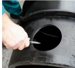
Clean the borehole
