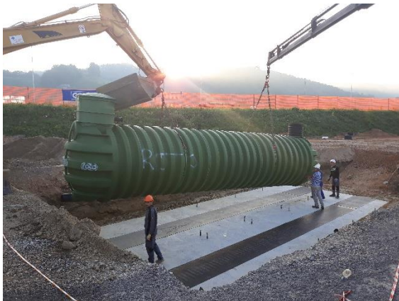
Picture 4: Installing the tank
