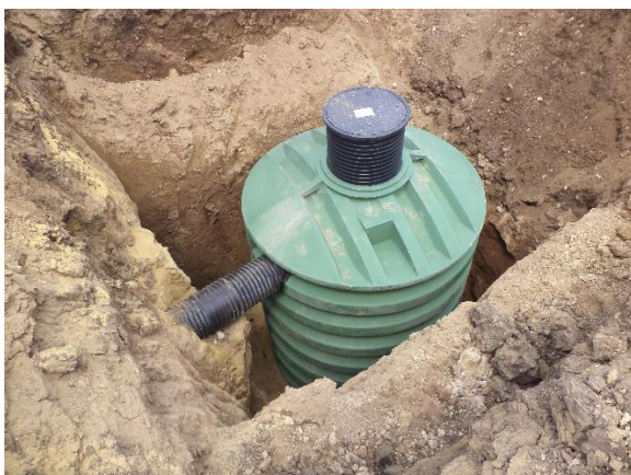
Picture 6: Installed tank
