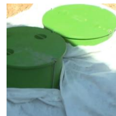
When the tanks are buried to the last 20 – 30 cm from the terrain lay down the geotextile
